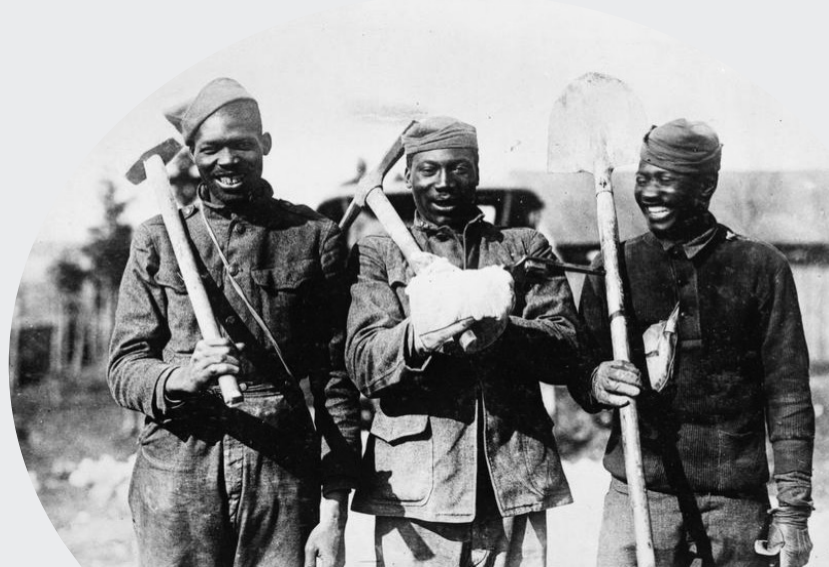
Black members of the US Engineers at Menil-LaTour, France, March 1918
